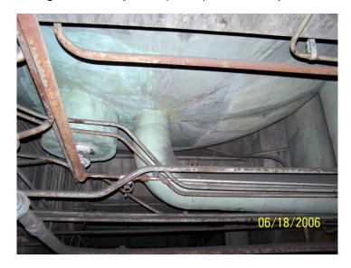
Figure 3: Underneath of Mercury Condenser Boiler
