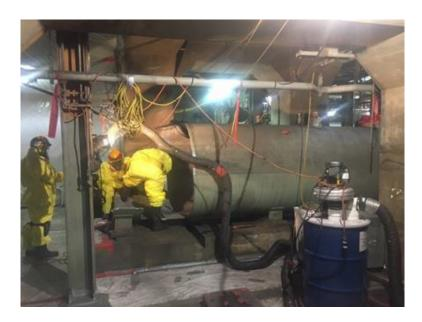
Figure 14: Removal of Mercury Storage Tank Through Non-Thermal Cutting
