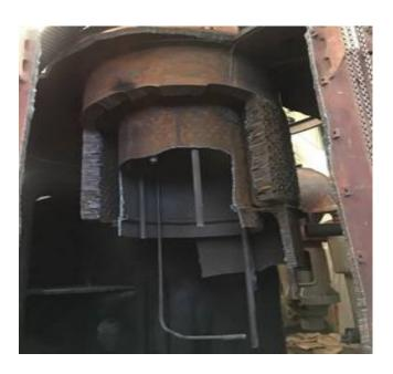
Figure 8: North Condenser, Turbine #1 (showing thickness of steel)
