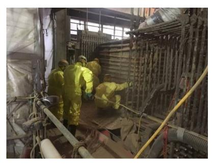
Figure 11: Unit 2 Removal of Boiler Tubes
