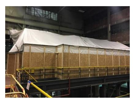
Figure 9: Containment over Turbine 1 and Associated Condensers
